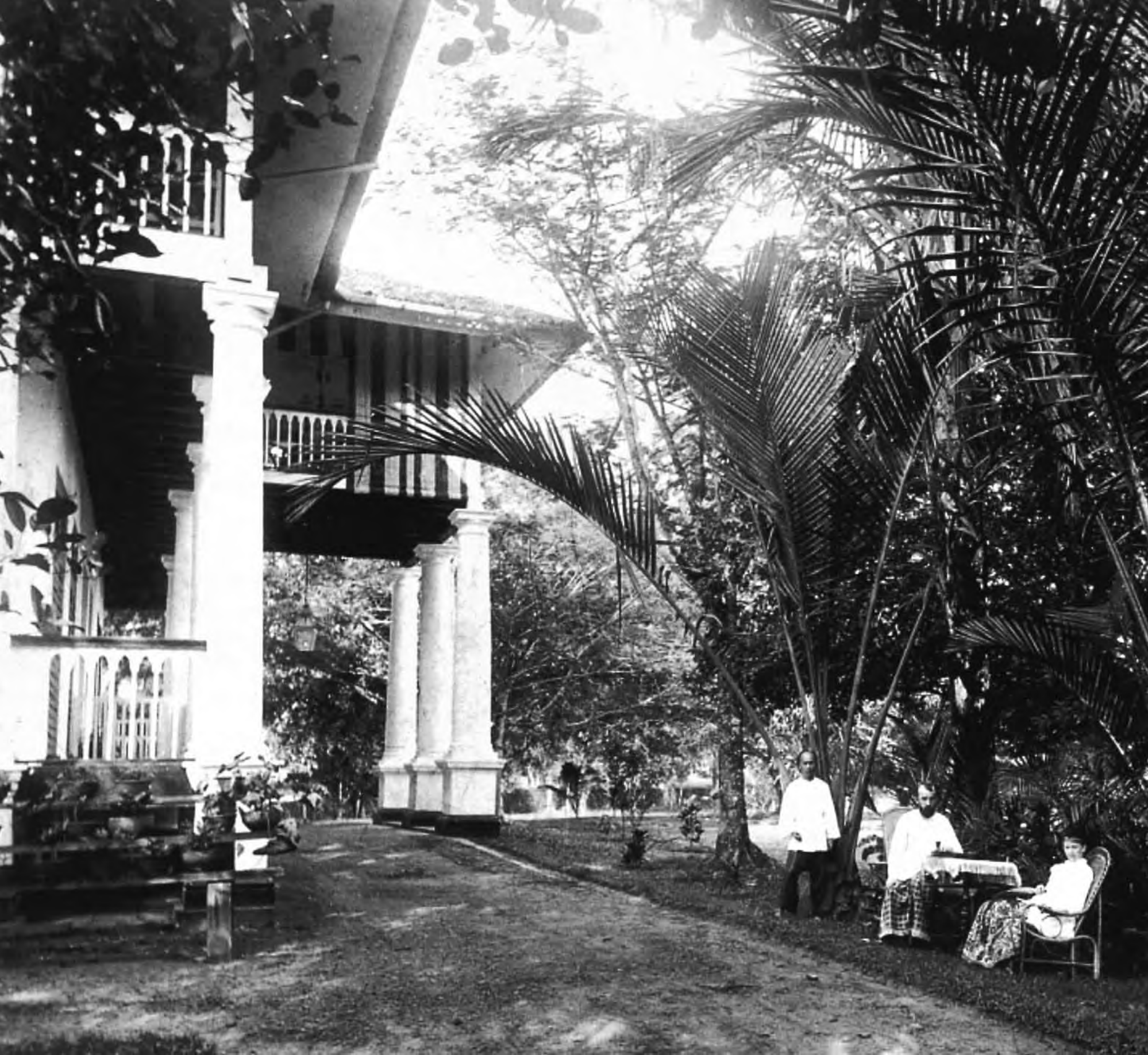
Colonial black and white house at Goodwood Hill
